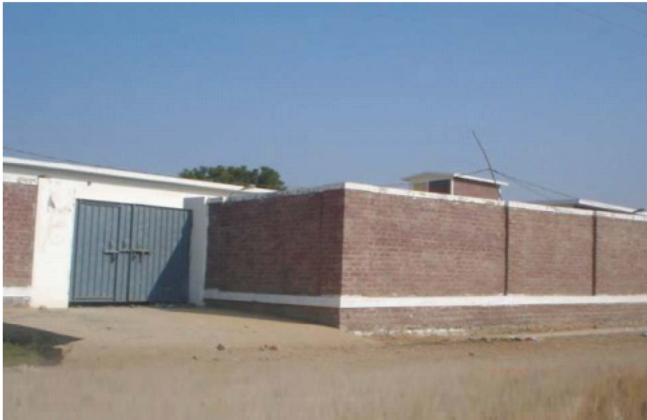
The Newly Constructed Building for Government Girls High School, Bhurgri
