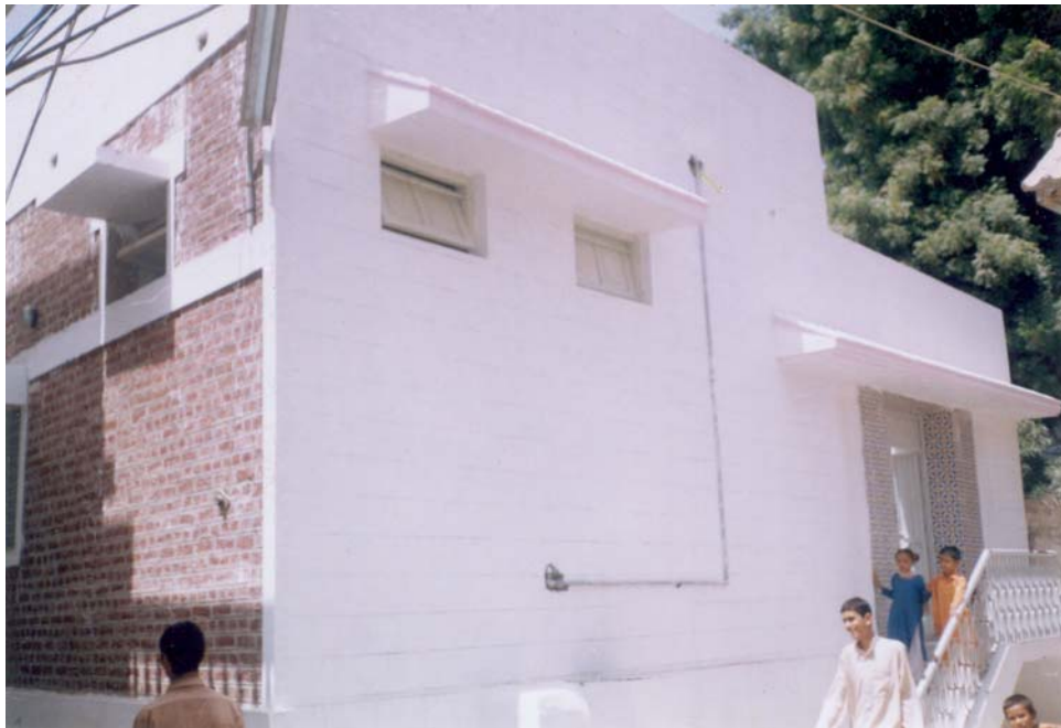
Main view of the school building
